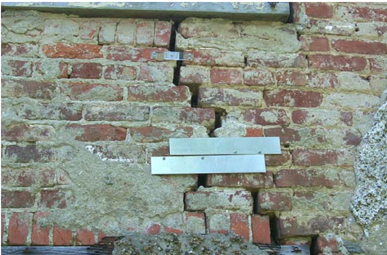
Typical Masonry Crack
